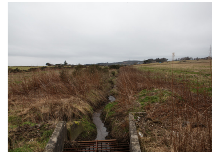
Typical watercourse character and outfall
